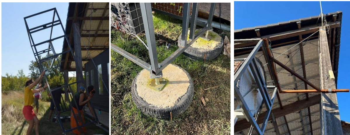
Figure 11. Installation des cages
